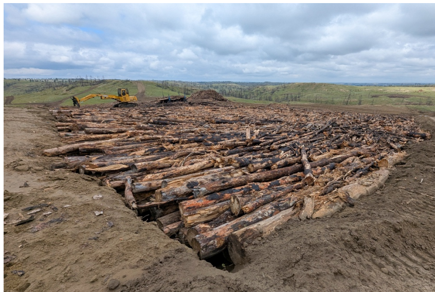
Figure 1: Mast Wood Preserve MT1 Chamber with Fire Damaged Trees
