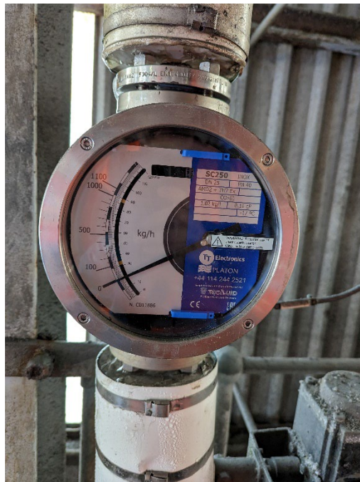
Figure A2-2. CO 2 injection flow meter at O.C.O Avonmouth
