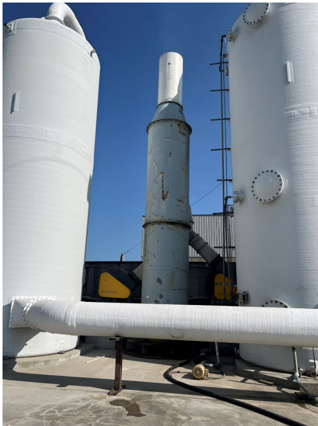
Figure A2-4. Venturi scrubbers (sides) and exhaust stack (middle)
