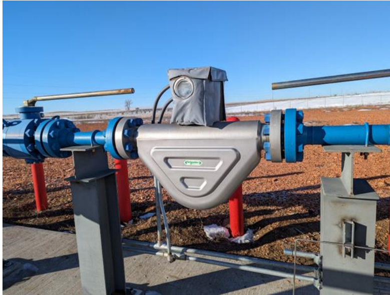
Figure A2-3. Calibrated Coriolis Meter at Injection Point
