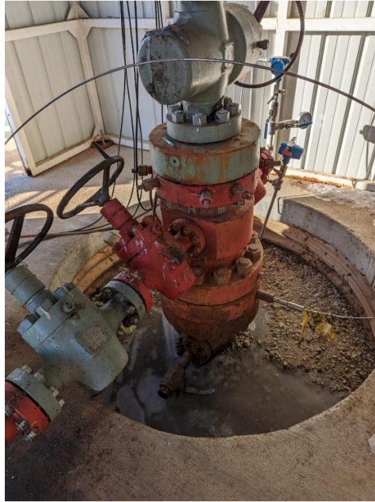
FIGURE 3. RED TRAIL ENERGY CO 2 INJECTION WELLHEAD
