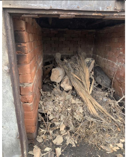
Reactor made from steel material mostly with alls of the reactor covered by of normal bricks
