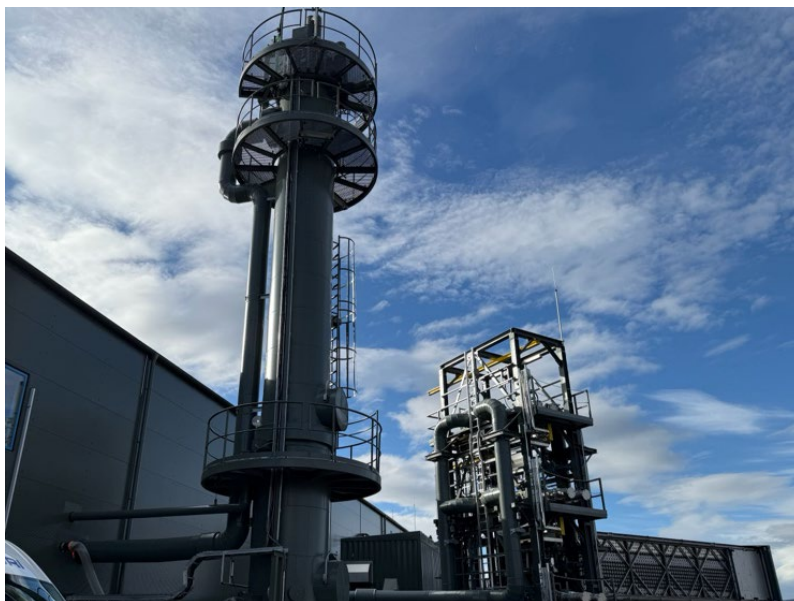
Figure 4: Absorption tower where the captured CO 2 is dissolved into treated water.
