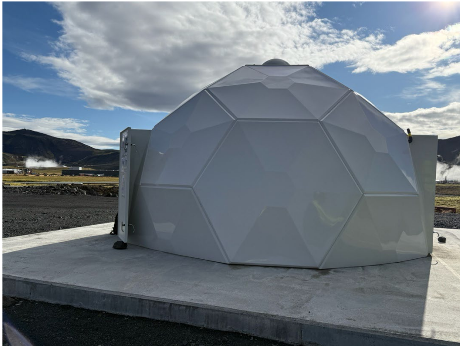
Figure B: Carbfix CO 2 charged water Injection well housing, one of two.
